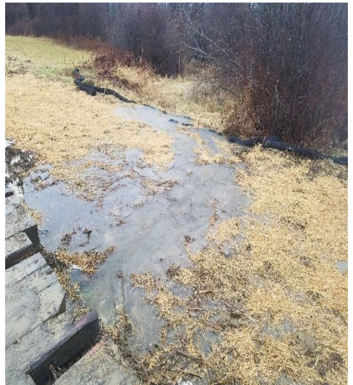
Fig 8: Wetland NW18 at Frink farm. Filter sock not installed correctly. Viewing north. (12-14-19).
