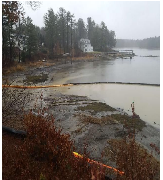
Fig 4: Most of the sediment being contained by the turbidity barrier at Gundalow landing/east side of the Bay. Viewing south. (12-14-19).
