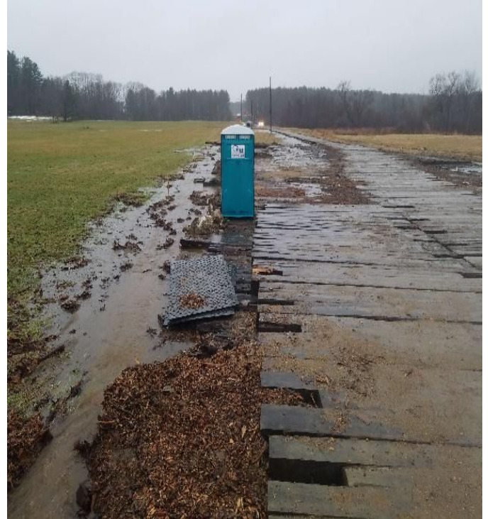
Fig 6: Runoff from Nimble Hill Rd through Frink farm. Viewing west. (12-14-19).
